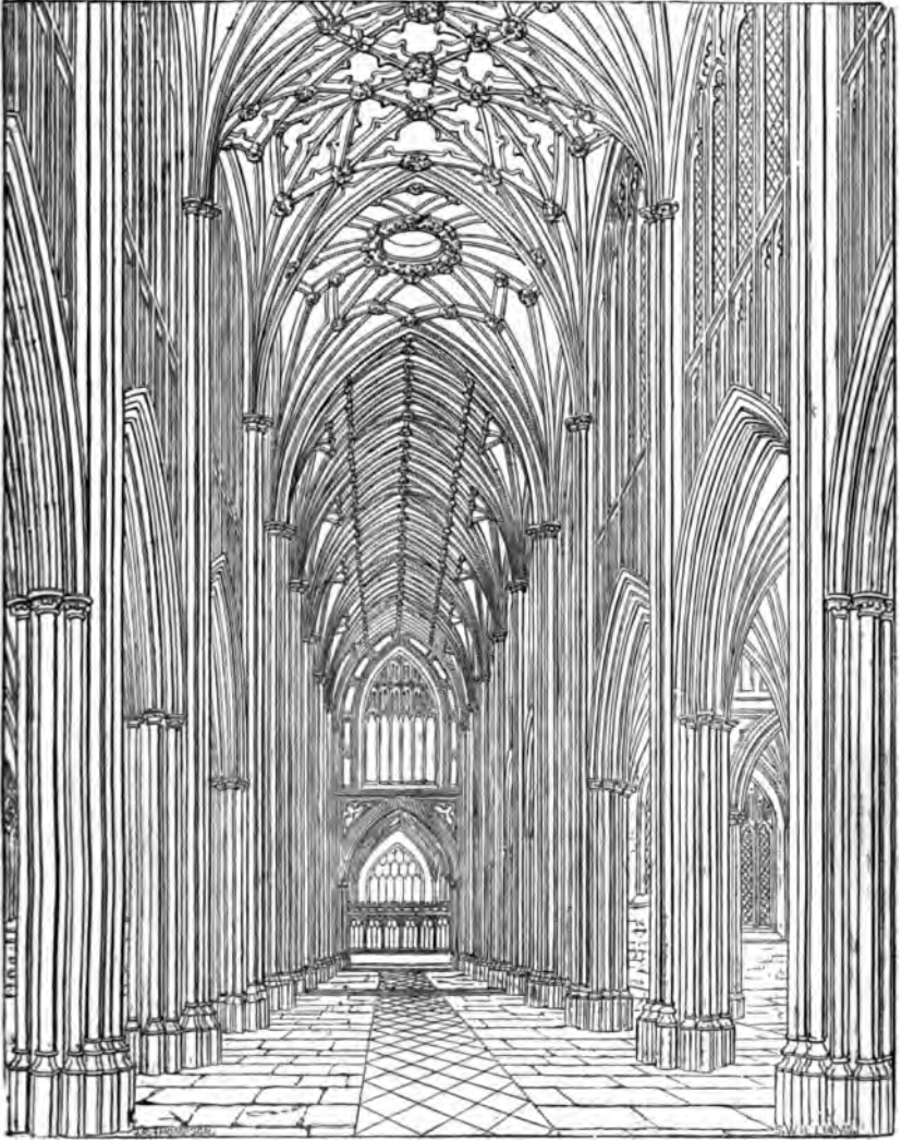
ST. MARY REDCLIFFE, BRISTOL. (Interior View, Restored.)
